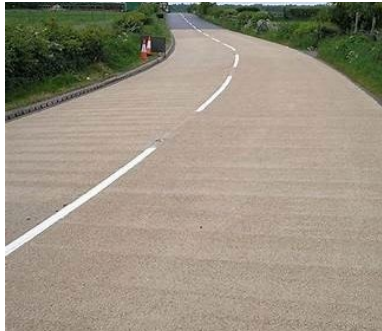
High Friction Surfacing on Road
