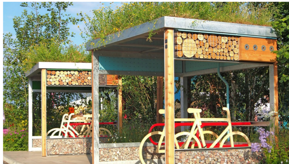
Green roofs can provide stepping stones of green infrastructure.
