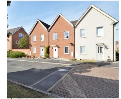
Block sett paving to junction: Tertiary
