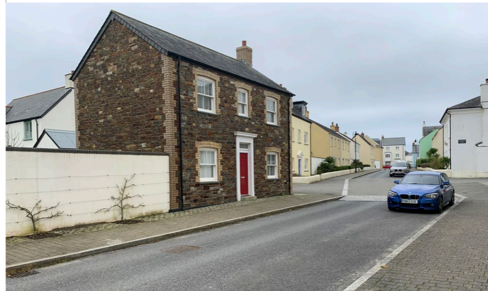
Nansledan, Newquay - use of nodal building and alignment change to slow traffic
