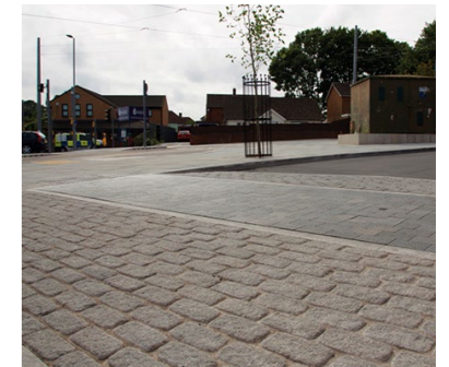
Setts with Asphalt
