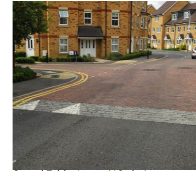
Speed Table Across Whole Junction
