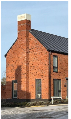
Chimney as an integrated part of the built form.
