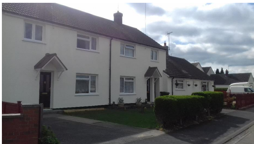
Completed External Wall Insulation – Long Lawford
