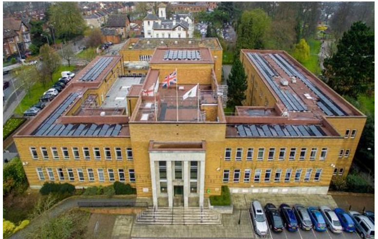
Rugby Town Hall Completed Solar Panel Project
