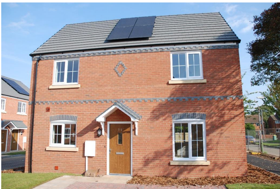
Completed Affordable Housing Pettiver Crescent, Hillmorton
