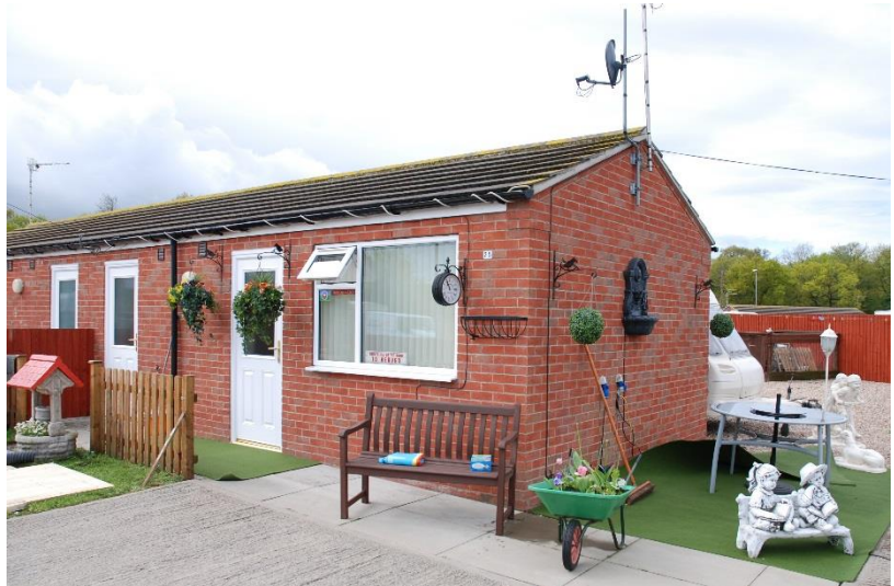
Completed Plot at Woodside Park Gypsy and Traveller Site, Ryton-on-Dunsmore
