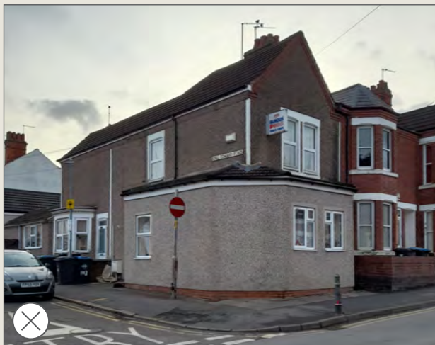
Above and above right: These examples do not represent high quality proposals for the residential conversion of shopfronts. They do not retain an active relationship to the street, no shopfront features have been retained and the placement and proportions of new windows and doors do not appear to have been considered within the building as a whole.
