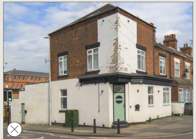
Above and above right: These examples do not represent high quality proposals for the residential conversion of shopfronts. They do not retain an active relationship to the street, no shopfront features have been retained and the placement and proportions of new windows and doors do not appear to have been considered within the building as a whole.
