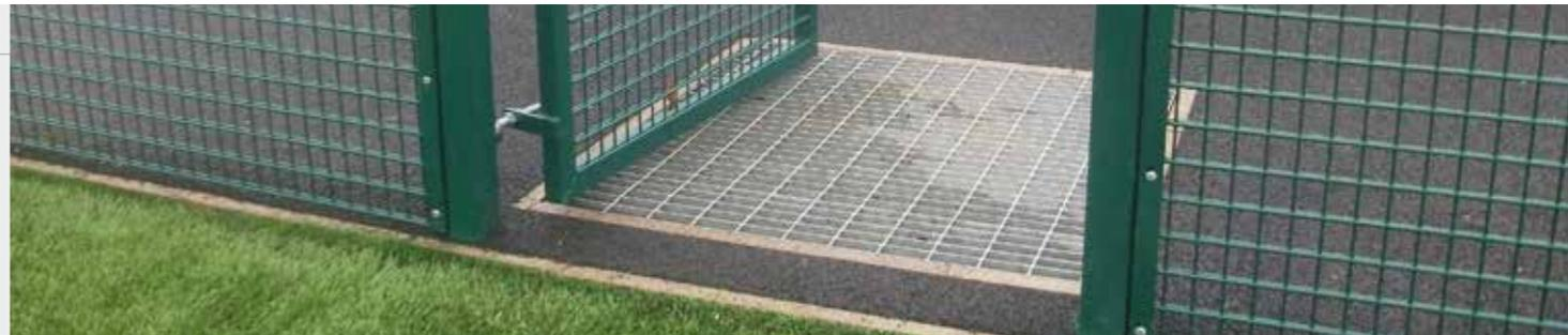
The access pathway to a 3G FTP should be fenced to ensure players and spectators don't walk debris onto the pitch.
